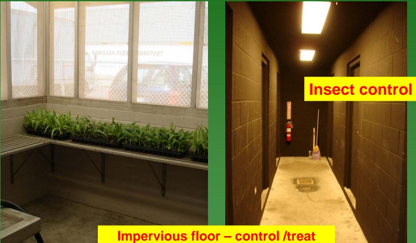
mpervious floor – control /trea water runoff
